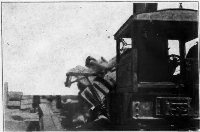
Discharging Stone Into the 60 Inch Crusher
